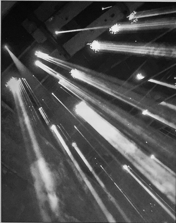
Bullet and shotgun holes had destroyed the roof, albeit artistically.
