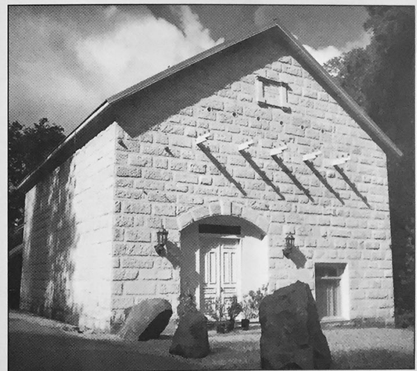
The mighty Utica Powerhouse is no longer an eyesore and once again graces the side of Utica Powerhouse Road in Murphys.
